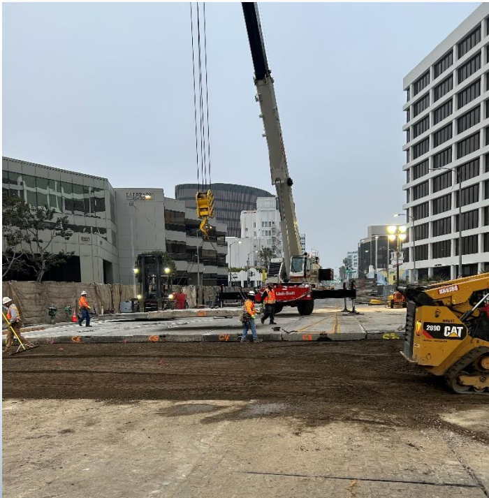
Backfill beneath deck panels
