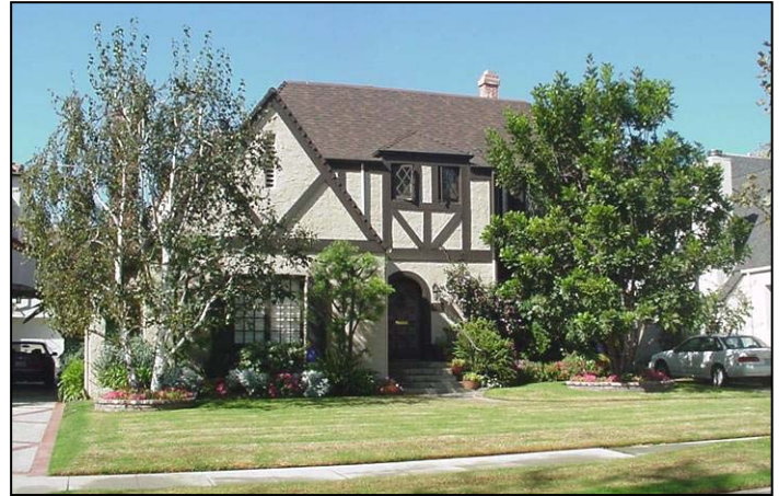
Photograph illustrates proportions of windows, roof pitches, and details associated with the style. Residence in photograph is located on a property approximately 60 feet in width.
