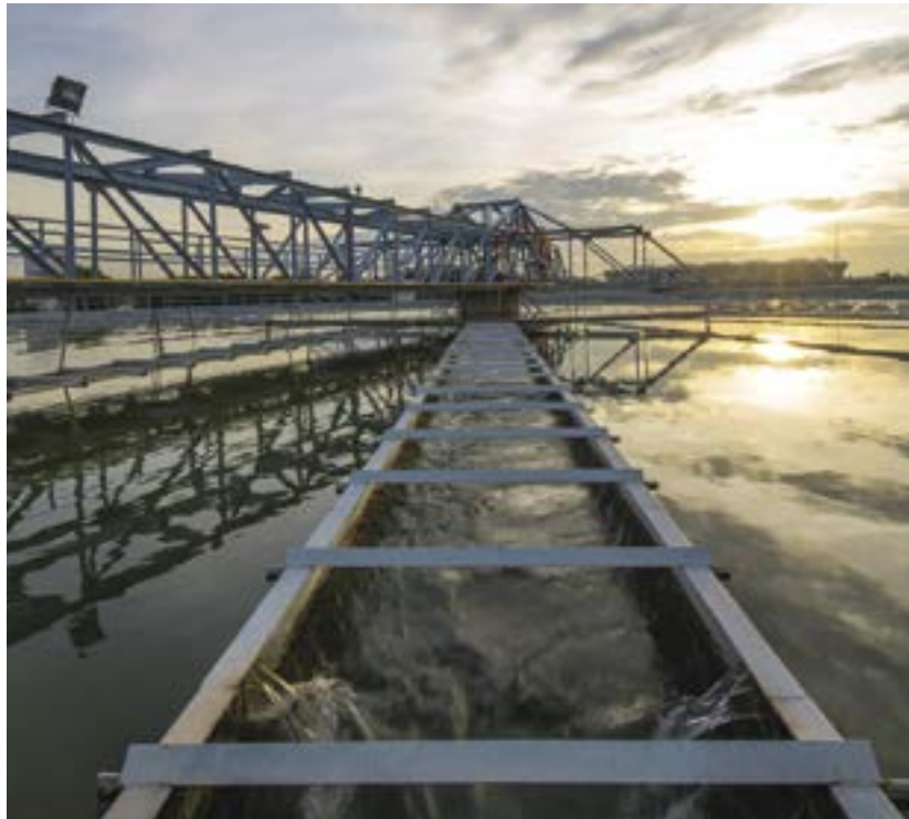
Jensen Treatment Plant
